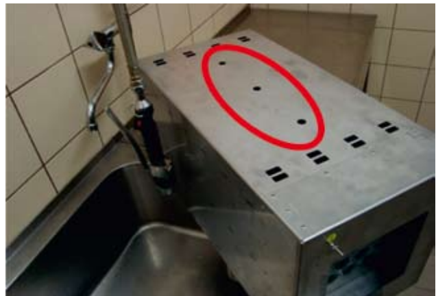
Picture 5 - Service openings
